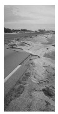
Texas road damage from flooding. Photo: FEMA
