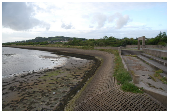
Image 1: An example of concrete revetment along a riverbank
